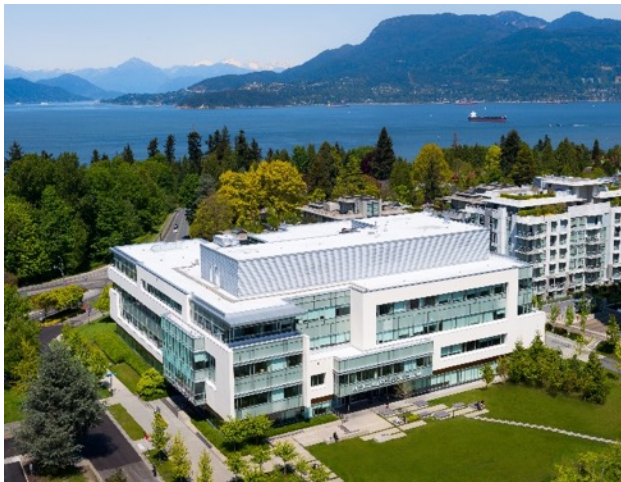
Allard Hall, University of British Columbia 1822 East Mall, Vancouver
